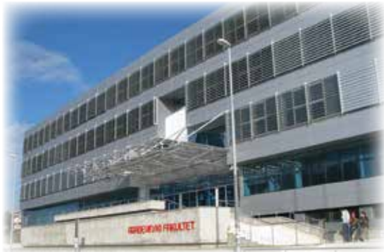
/Photo: Faculty of Civil Engineering, Faculty archives/
